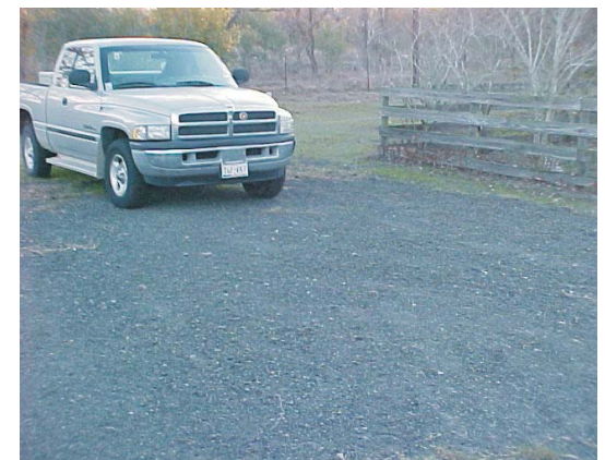
Local driveway topped with Washed Bottom Ash
